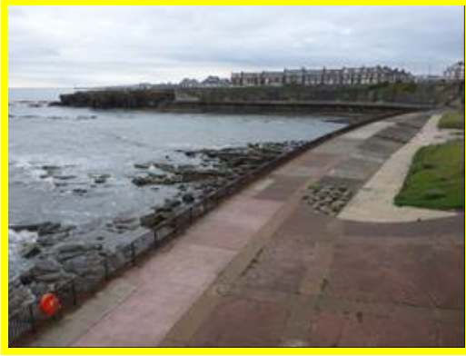
Brown's Bay northern sea wall in generally fair condition (/4601C10)
