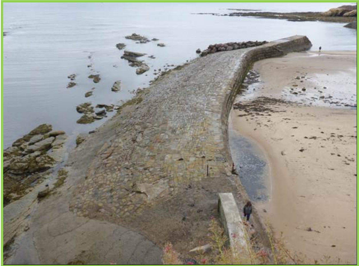
Cullercoats North Pier in good condition following repair works (I4701C07)
