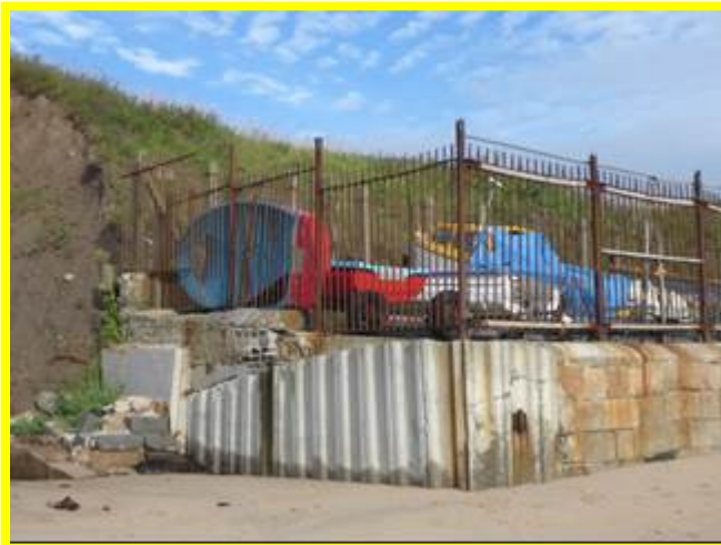
Wall at boatyard (/4501C05)
