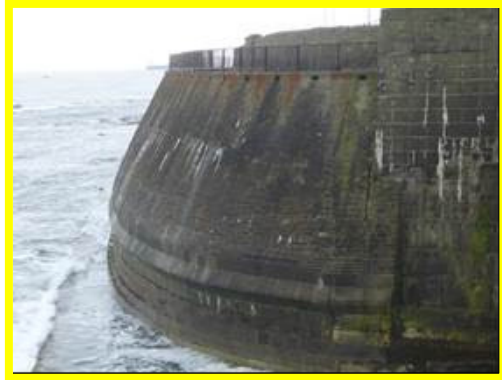
High blockwork sea wall (/4601C06)
