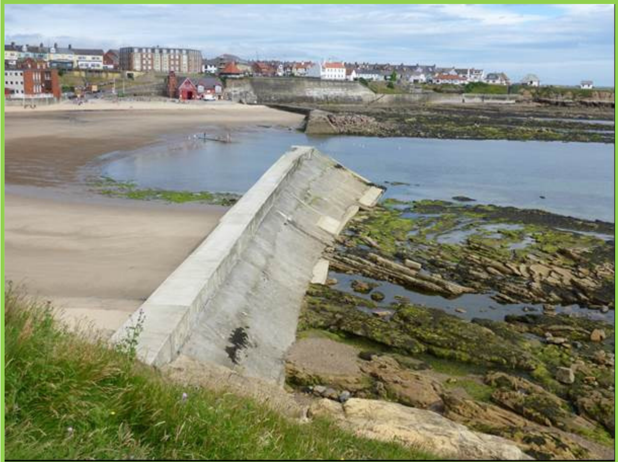
Cullercoats South Pier in very good condition following refurbishment works (/4701C15)
