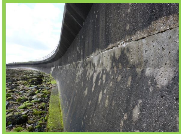
Trinity Road seawall in good overall condition, note the construction joints (/4501C04)
