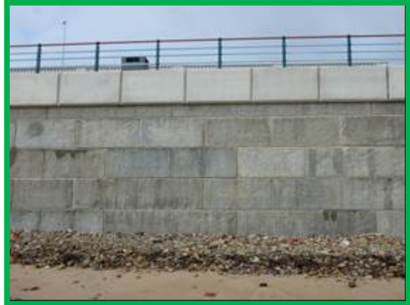
Refurbished sea wall (/4601C03)
