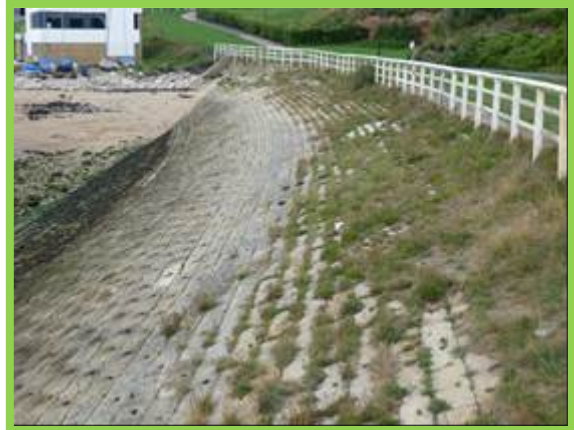
Masonry revetment (/4801C02)
