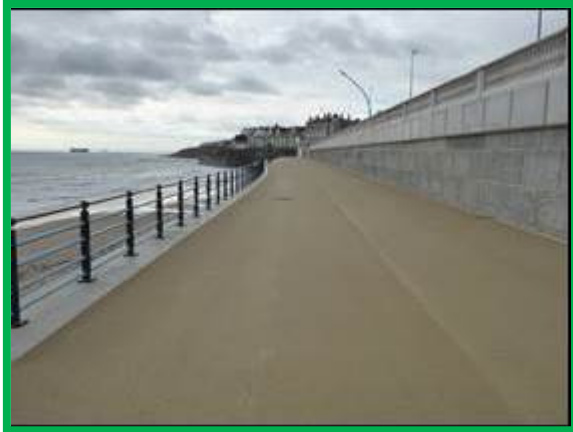
Refurbished promenade (/4601C03)
