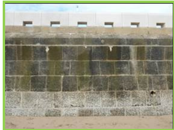
New coping on seawall (/4501C07)
