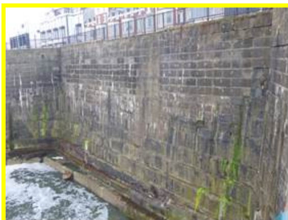
High blockwork sea wall (/4601C05)
