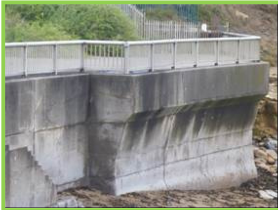
First section of sea wall in generally good condition (/4701C04)
