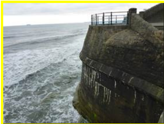
Blockwork sea wall at first 'bullnose' (/4601C04)
